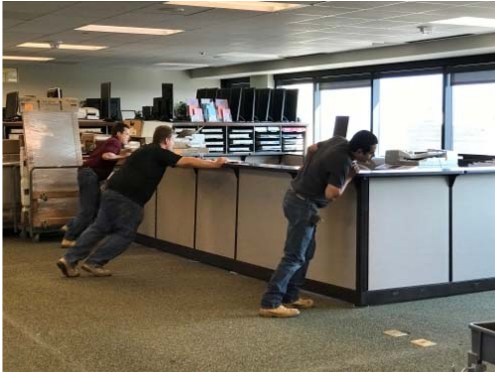
office renovation underway
